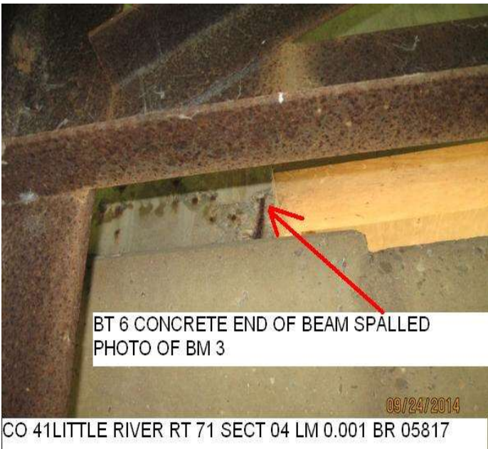
PHOTO 4 Description BENT 6 END OF BEAM
