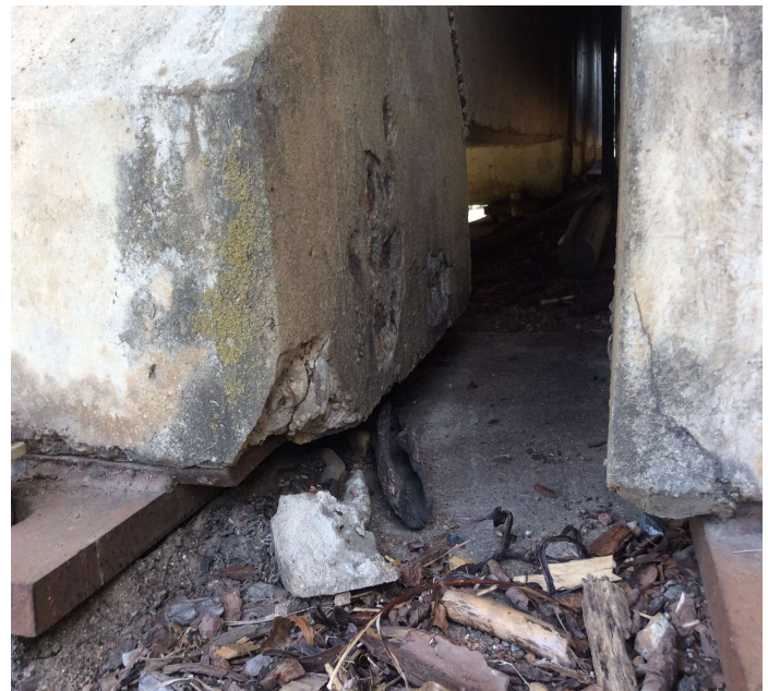
PHOTO 2 Description BENT 15 SPALLS AT BEARING AREA BEAM 3,4, AND 5
