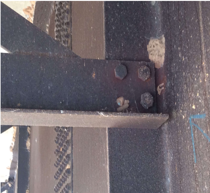
PHOTO 1 Description 1 missing bolt and 1 loose bolt beam 2 bay 1 span 9 2nd crossbrace in span 9
