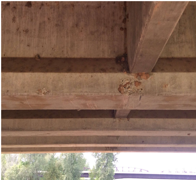
PHOTO 1 Description SPAN 5 BEAM 4 SPALL
